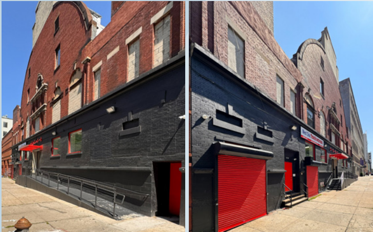
View along West 124th Street - ADA Accessible Ramp from sidewalk
