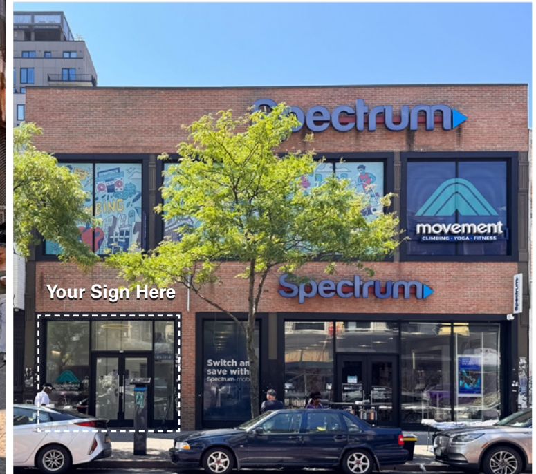
View of direct 125th Street entry via elevator or stairway through shared lobby with Movement Harlem
