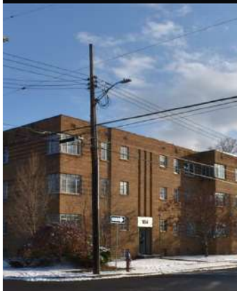
2. 162 CHAPIN STREET Binghamton, NY 13905
