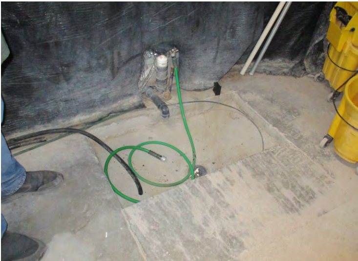
Photo 41 - View of a floor drain in Greenhouse 1.
