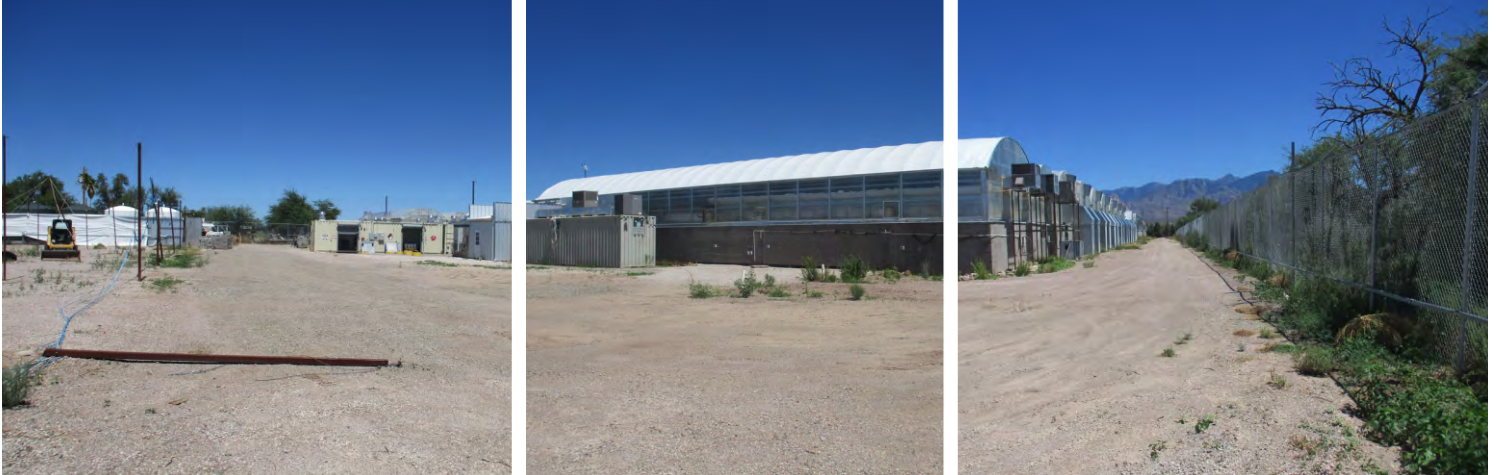
Photos 4, 5, 6 - View of the subject property, looking north, northeast and east from its south fence west of Greenhouse 1.
