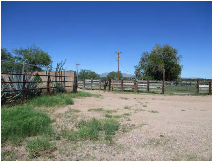
Photo 45 - View of the north adjoining corrals, looking north through the subject property's northeast gate.
