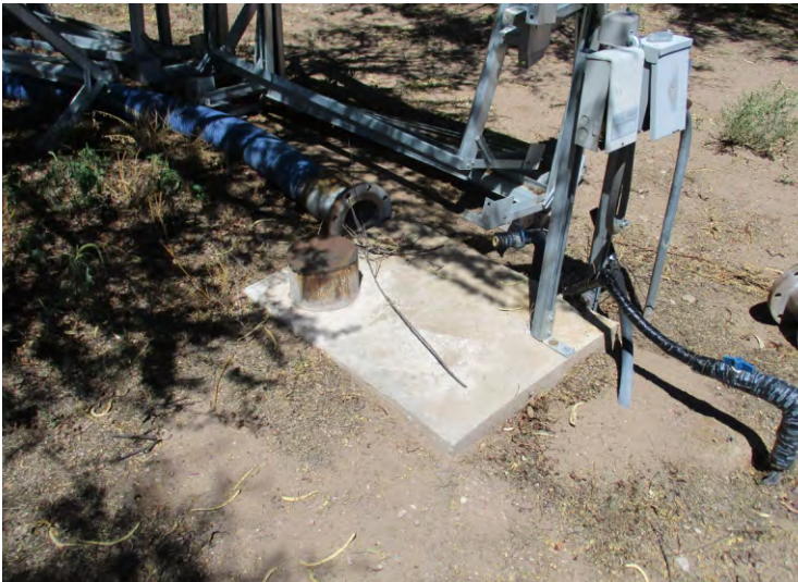
Photo 23 - View of the capped domestic well west of the ranch house.
