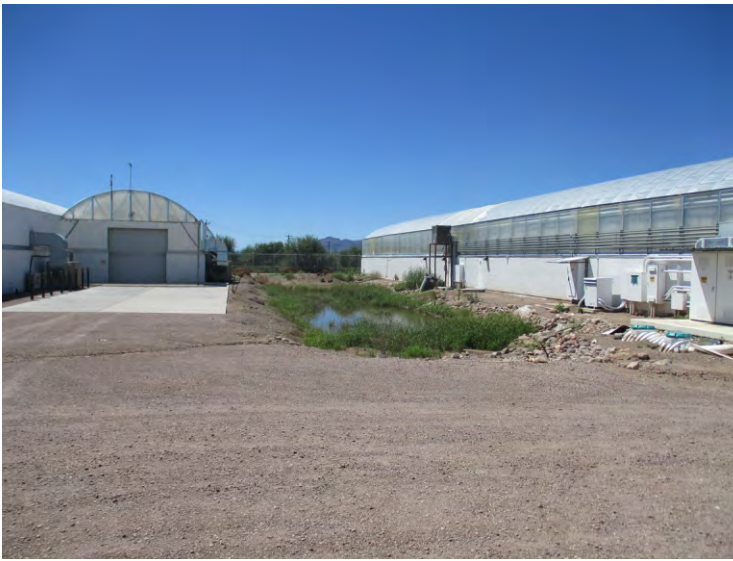
Photo 15 - View of the retention basin between Greenhouses 1 and 2, looking south.
