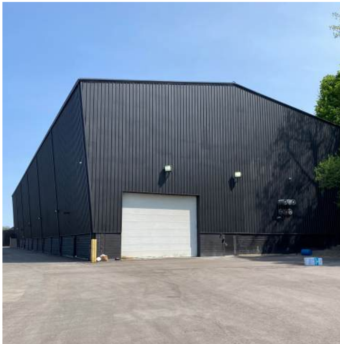
West Building - Mega Stage
