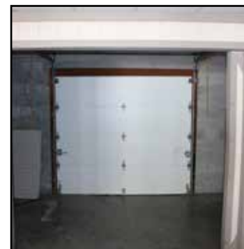
111: Roll-Up door in storage area
