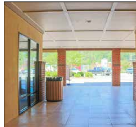
Breezeway, looking out toward parking lot
