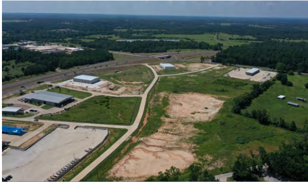
Aerial Photo Facing north along HWY 19
