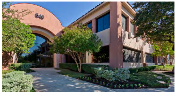
PLAZA II 540 OAK CENTRE DRIVE
