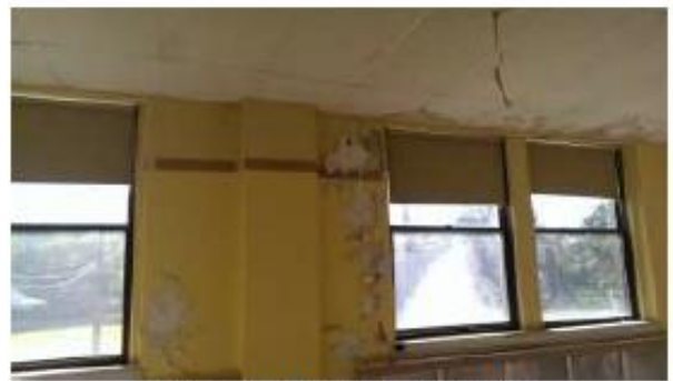
POSSIBLE WATER DAMAGE
