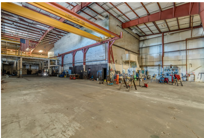
Clear-span warehouse with overhead bridge crane
