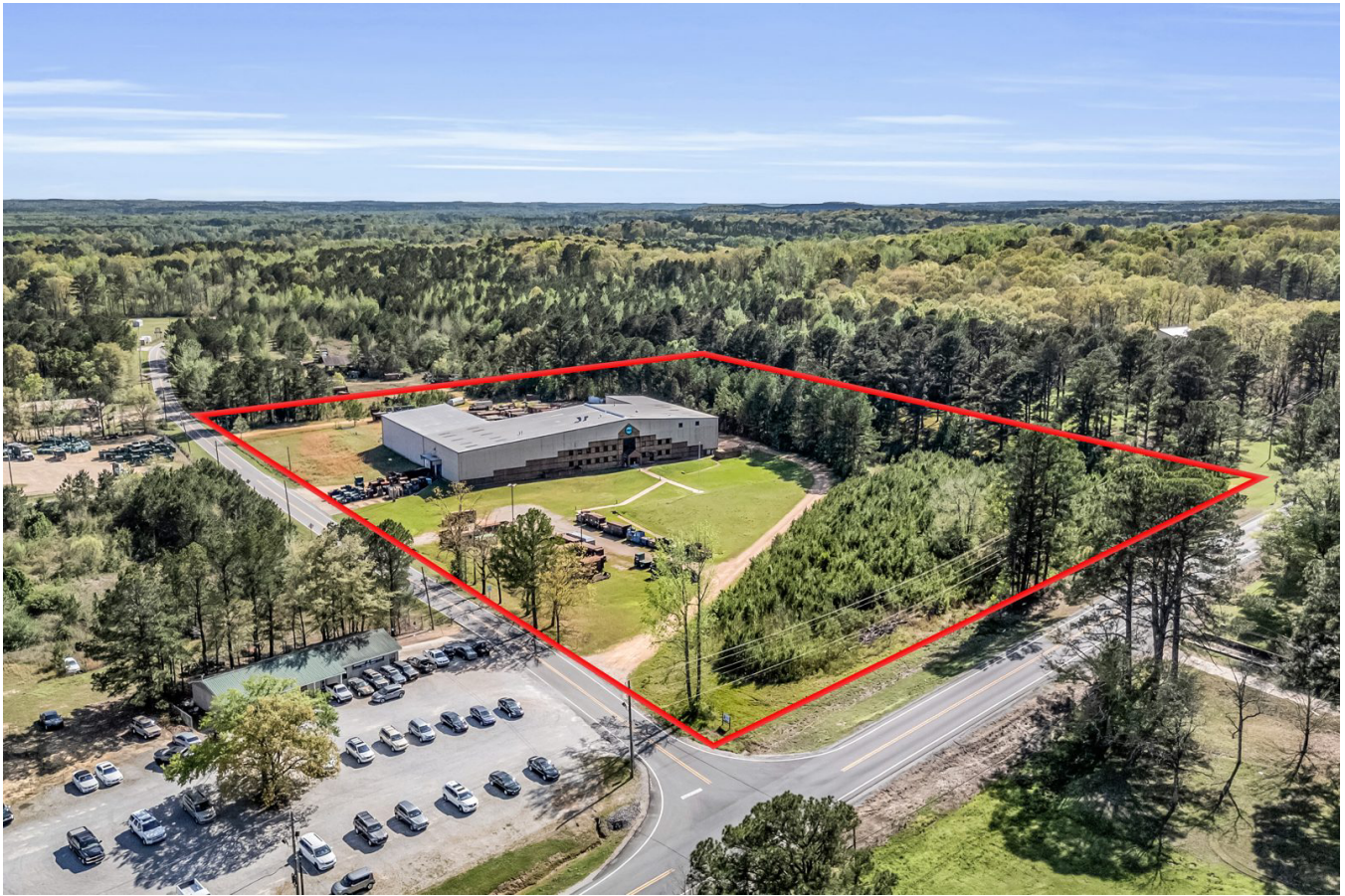
Aerial view with approximate 9.2-acre property boundary, fronting Highway 18.
