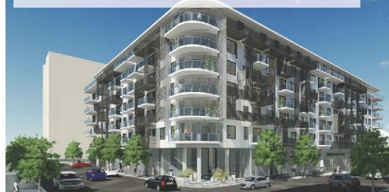
MODERA HOLLYWOOD 1546 Argyle Avenue
