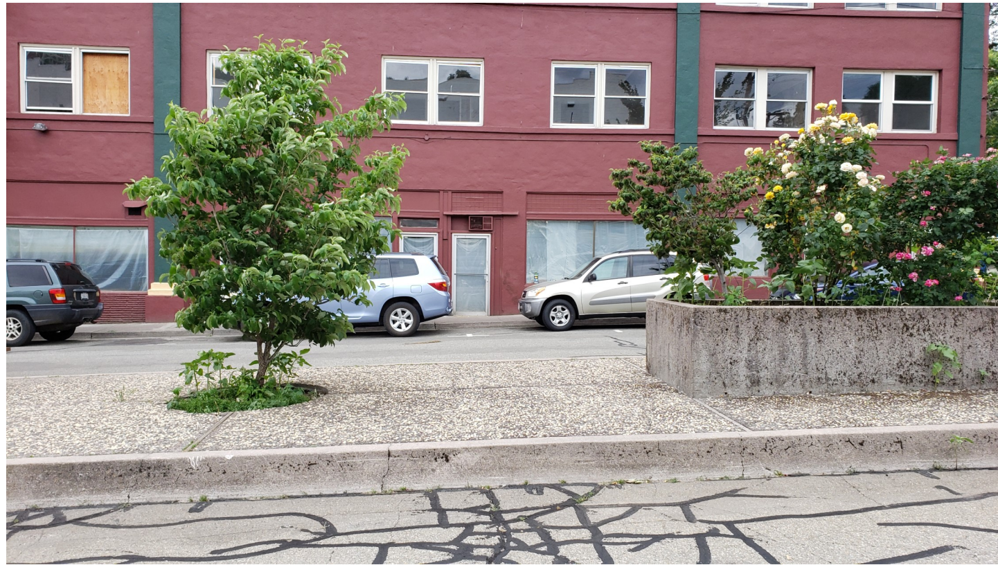
Existing Raised Island Median
