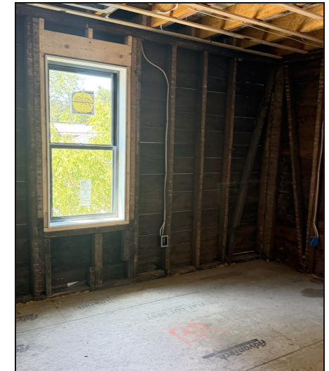
PEX supply & waste lines set
