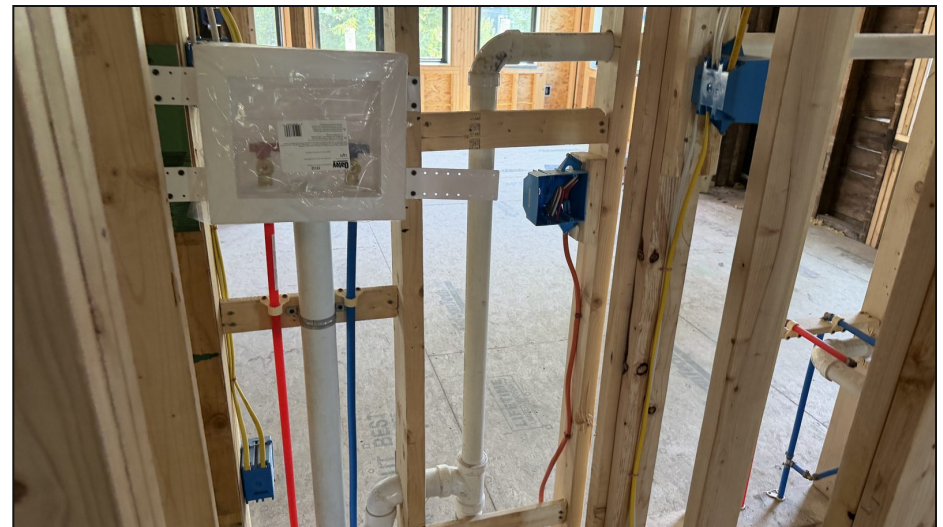
Bedroom framed with electrical rough-in complete
