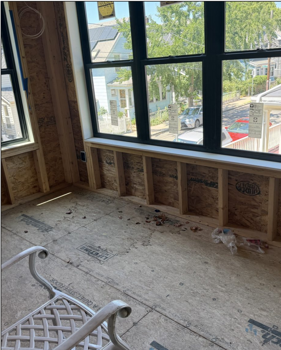
Oversized new thermal windows flood the principal rooms with light
