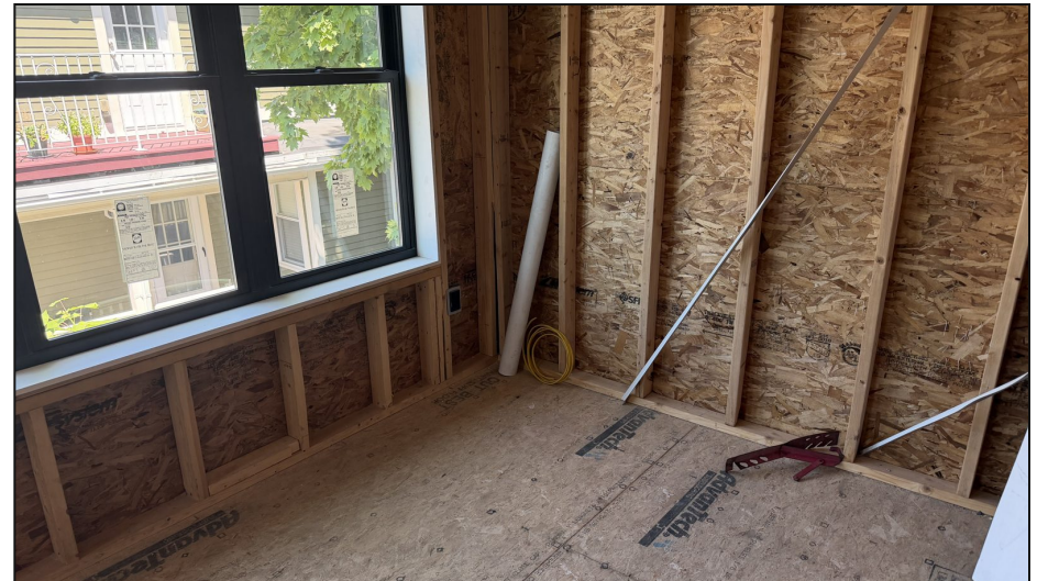
New framing and window packages throughout
