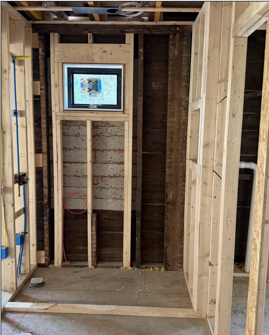
Wiring, ductwork and systems roughed through all four levels
