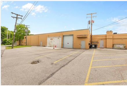
View of building exterior with central air condition unit
