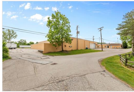
View of road
