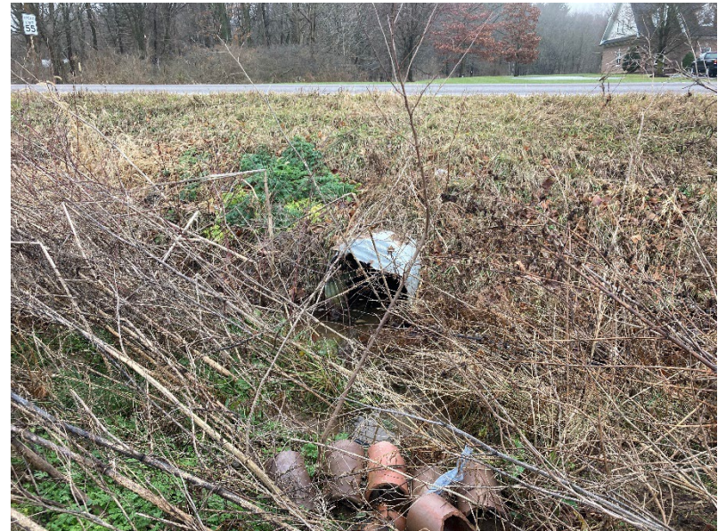
Photo 8: View of the culvert that carries roadside ditch hydrology downstream (east) under Coshocton Road.
