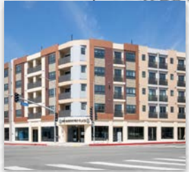
BARRINGWAY PLACE 11701 W Gateway Blvd
