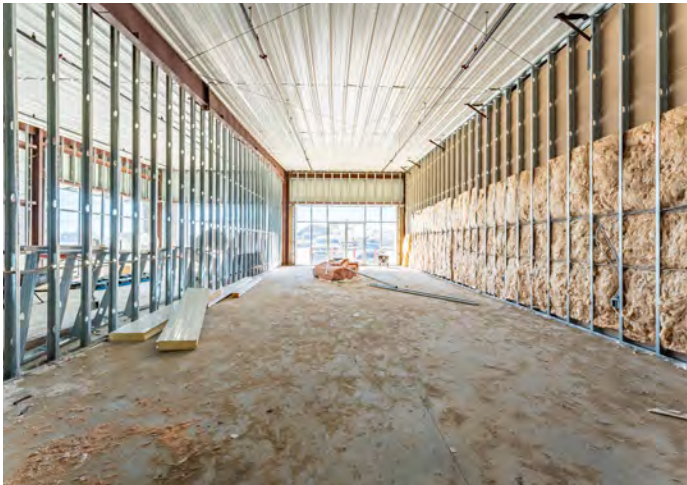
Shell Space Condition
