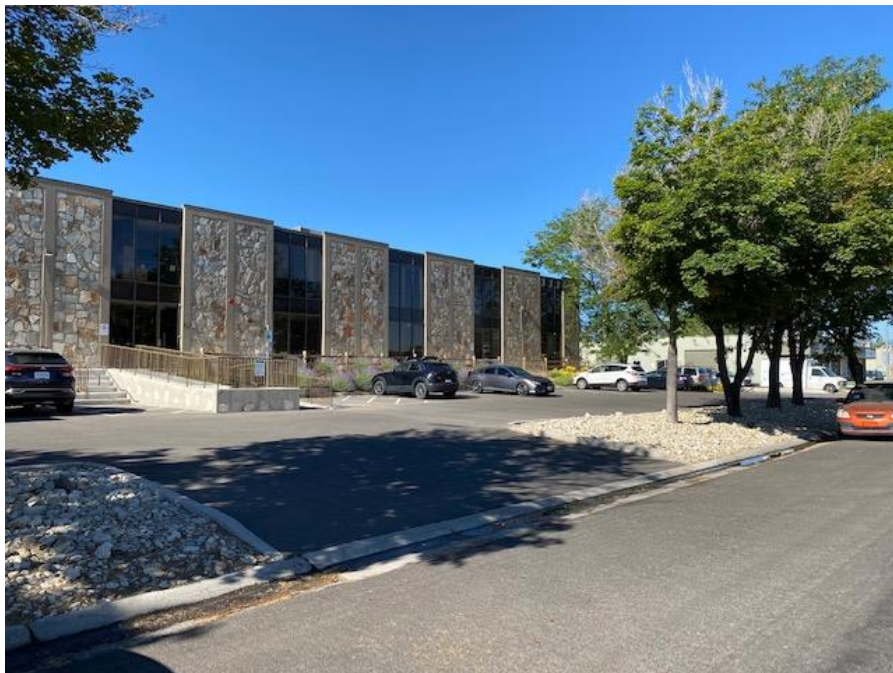
North Building Face Looking West
