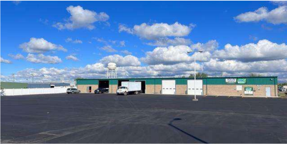
2 3241 E End Ave 3241 East End Ave South Chicago Heights, IL 60411
