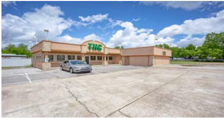
Front of building
