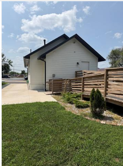
Back of Structure
