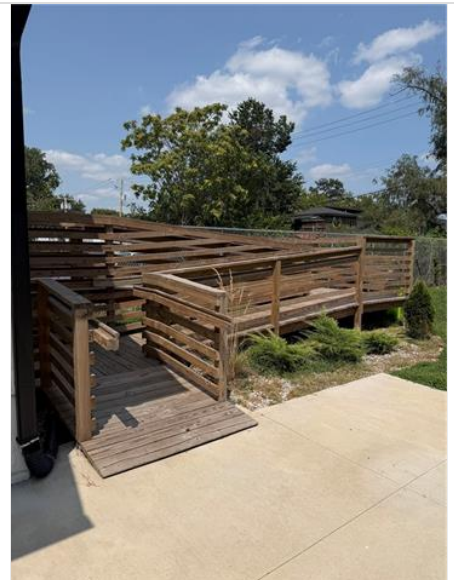
Accessible ramp from driveway to building.
