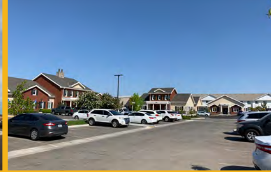
Hoffmann Hospice Free Standing In-Patient Hospice Facility, Administrative Building & Grief Support Building - 40,215 SF
