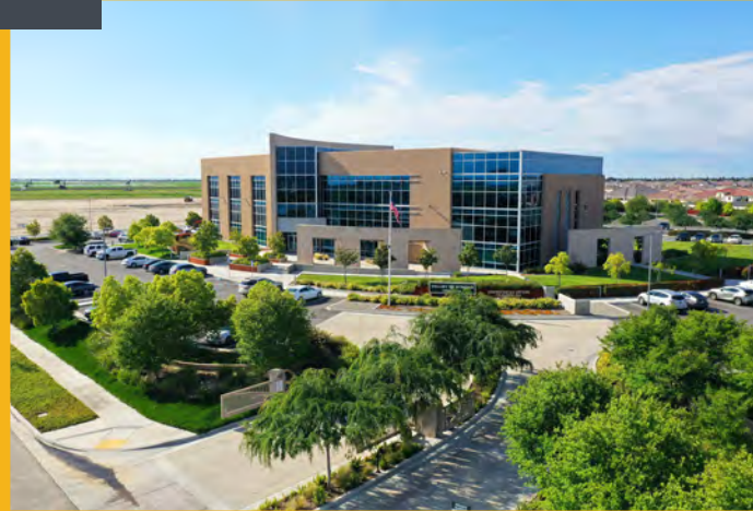
Valley Strong Credit Union 60,000 SF Headquarters
