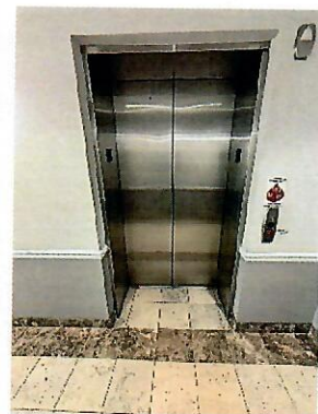
OTIS 3,000 lb. capacity elevator
