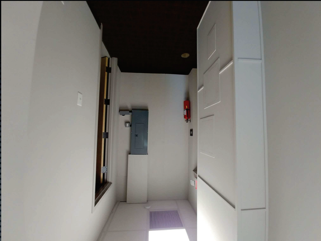
REAR EXIT CORRIDOR
