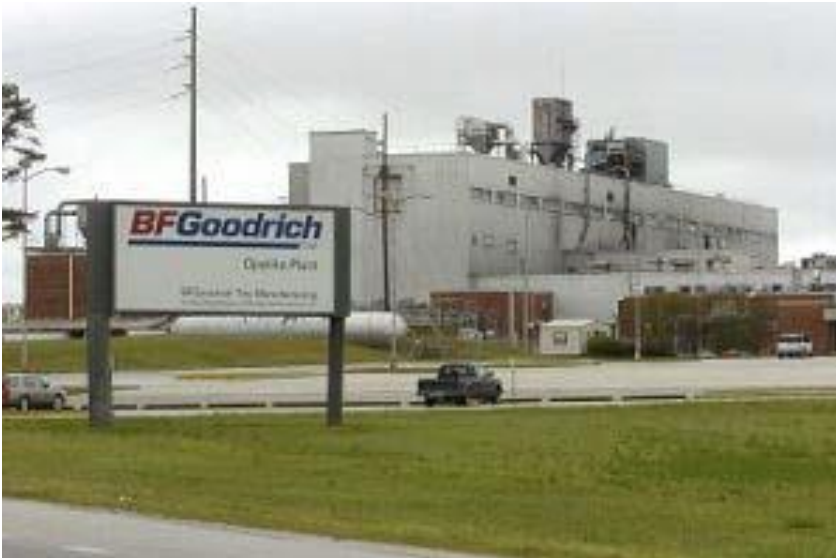
View of 3-Story Manufacturing Building
