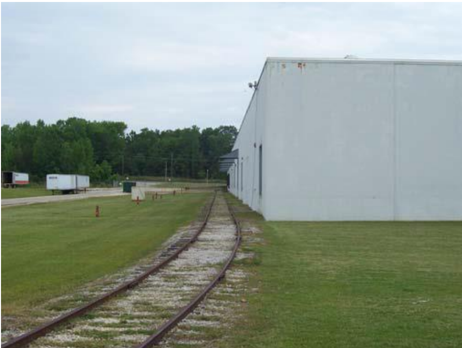
Rear Rail and Truck Loading Doors
