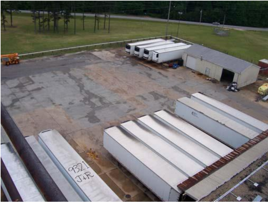
Front Receiving Area and View of Crawford Road
