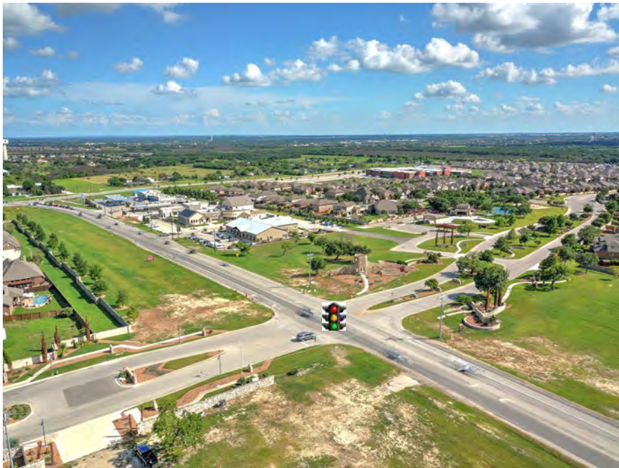
Intersection of FM 1103 and Turning Stone. Future Lighted Intersection
