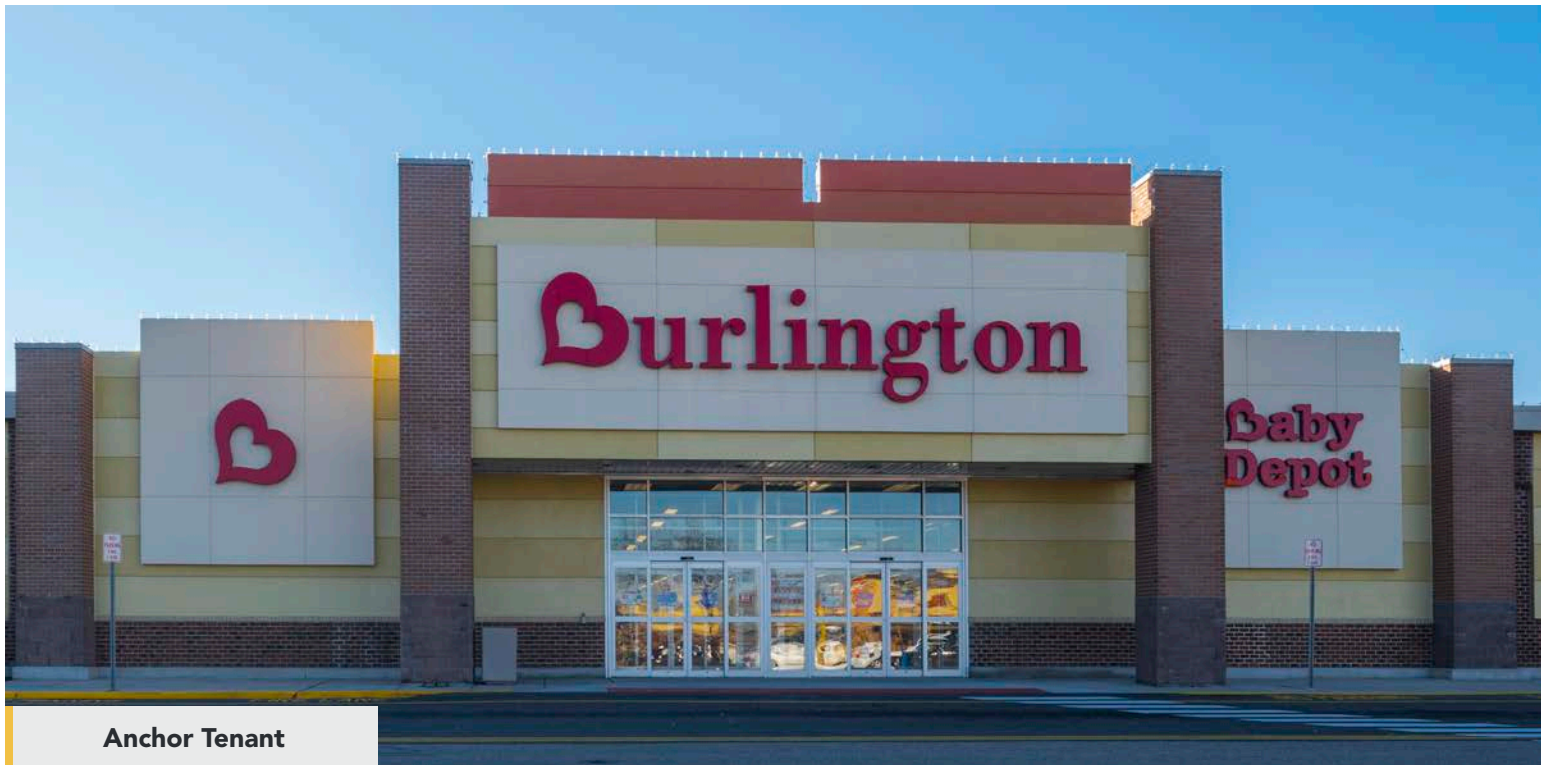
Existing Pad Building
