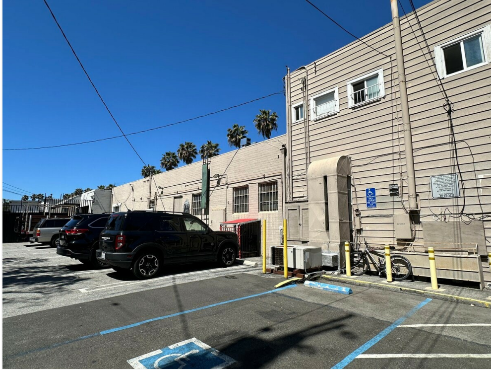
Rear parking lot
