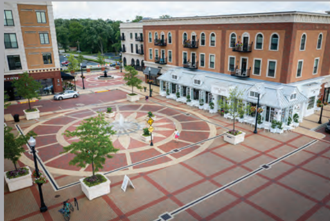
Plaza level photo of the United Fidelity Bank Building
