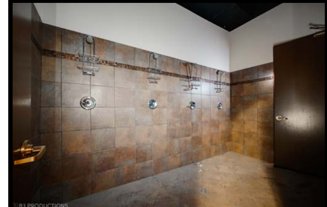
SEPARATE SHOWER AREA WITH 4 SHOWER HEADS ADJACENT TO LOCKER ROOM
