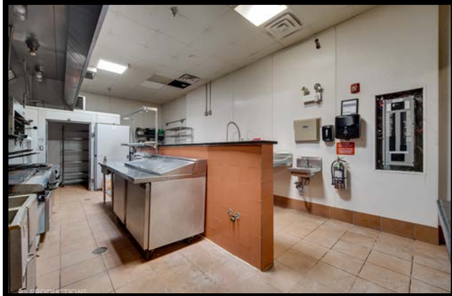
FULLY EQUIPPED KITCHEN WITH WIC, FRYERS, OVEN, STOVE AND STORAGE
