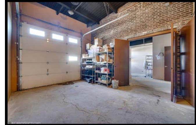
SECOND LOADING DOCK WITH EXTRA STORAGE
