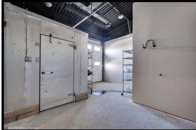
WALK-IN-FREEZER WITH LOADING DOCK
