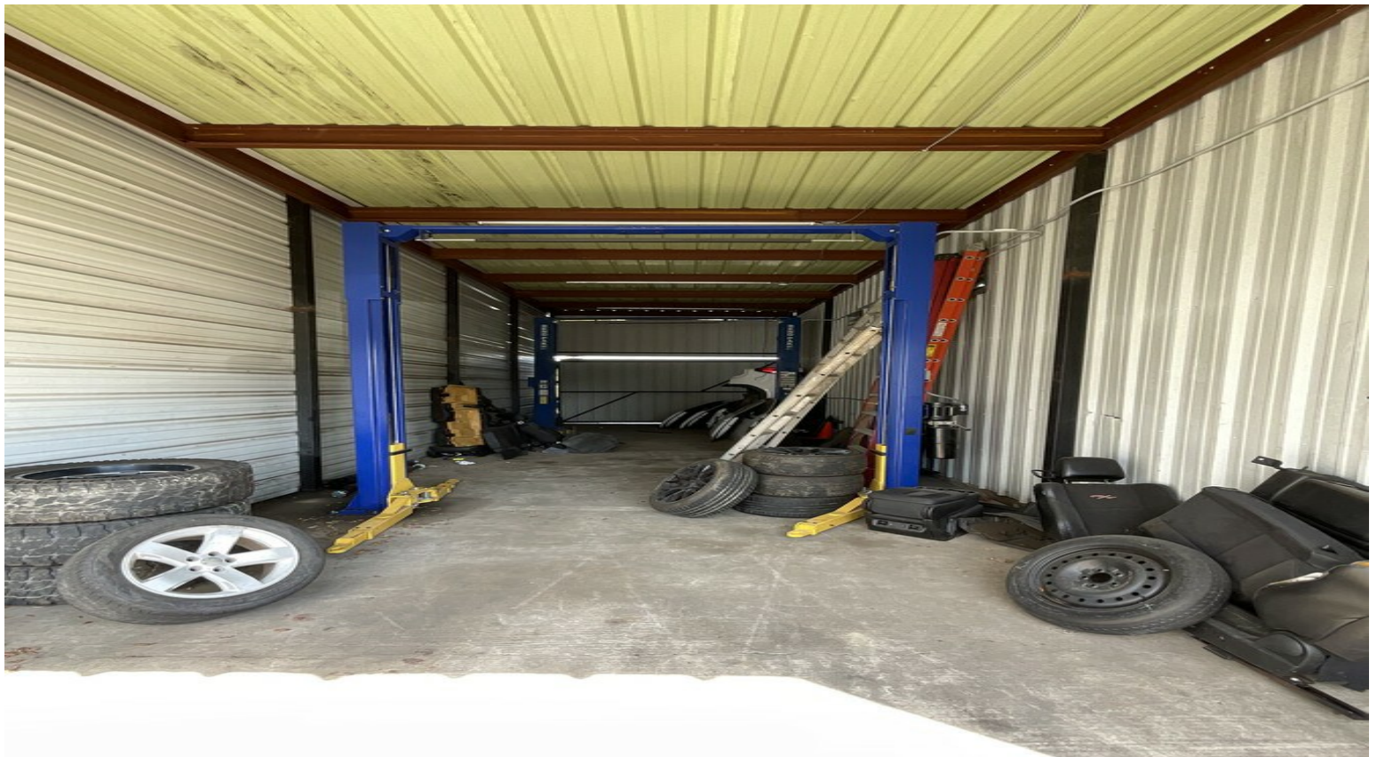
Photo of the secondary structure
