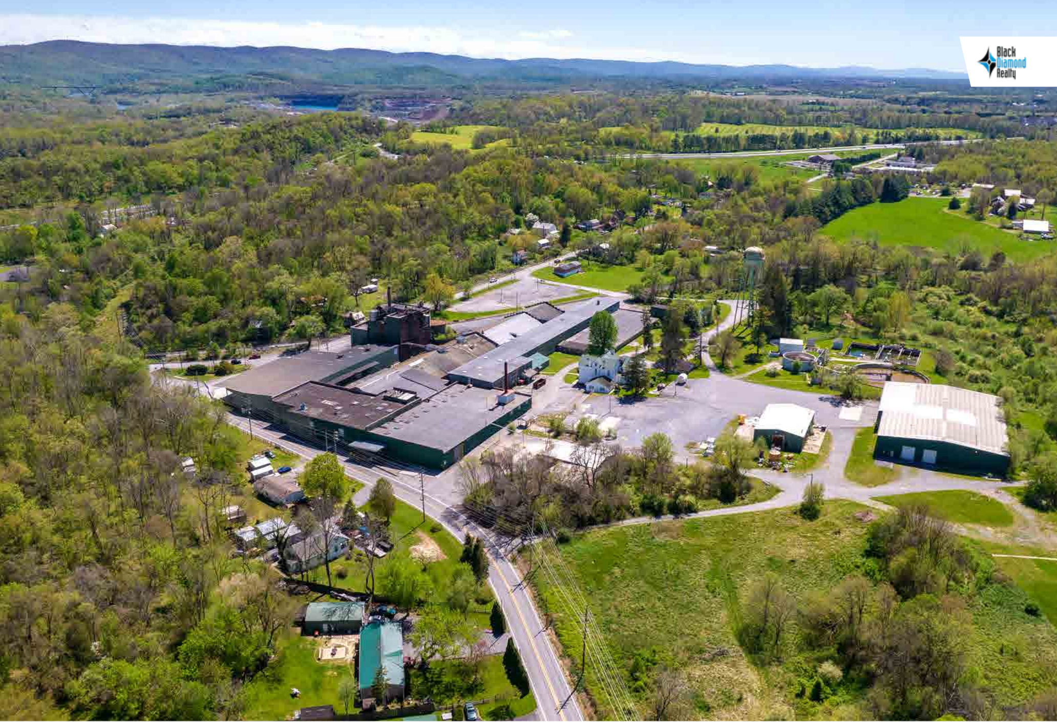
Aerial Facing South.
