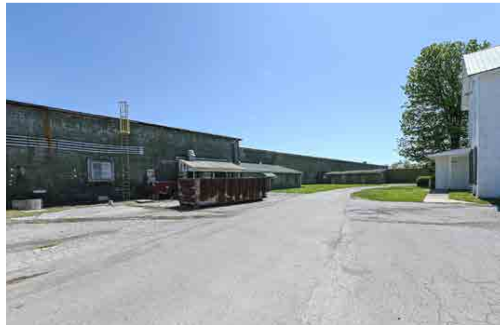
Property Exterior: Zone #1.
