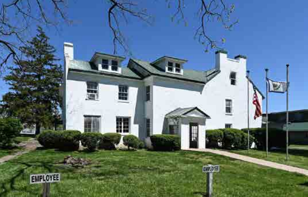
Admin House: Front Main Entrance.
