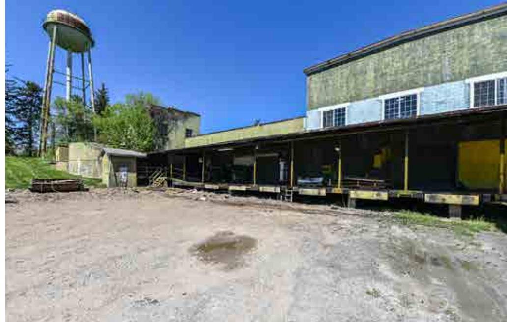
Property Exterior: Zone #9.
