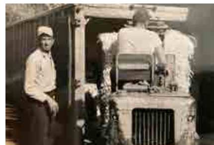
The mill has been focused on producing recycled paperboard since WWII
