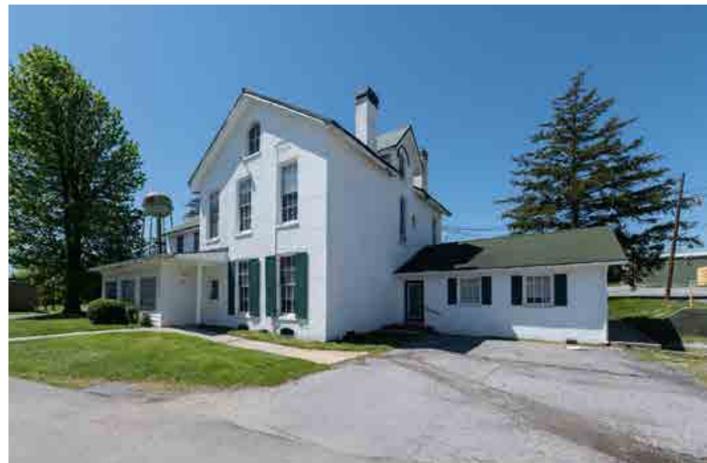
Admin House: Exterior.
