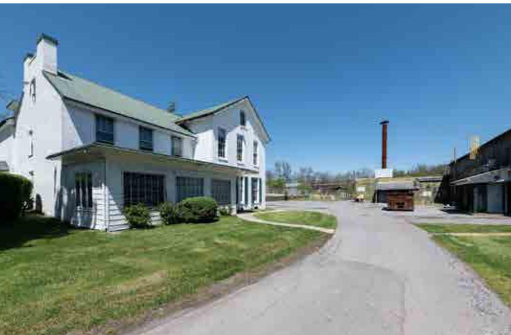
Admin House: Exterior.
