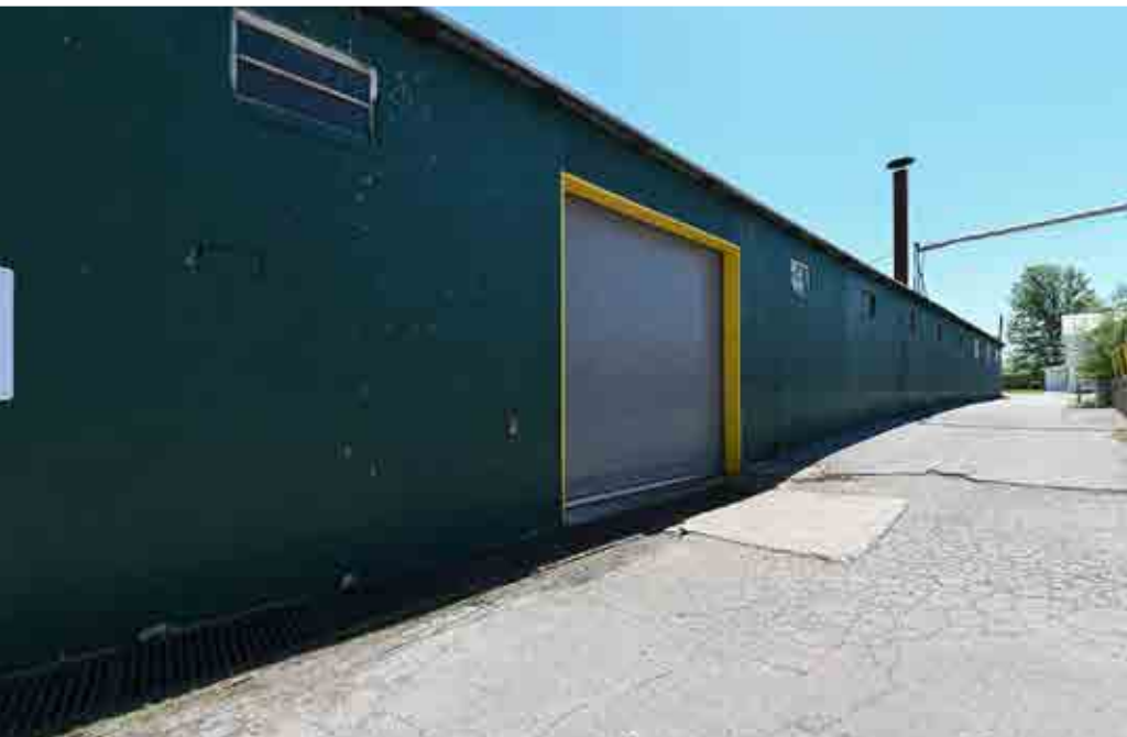
Property Exterior: Zone #8 & #4.
