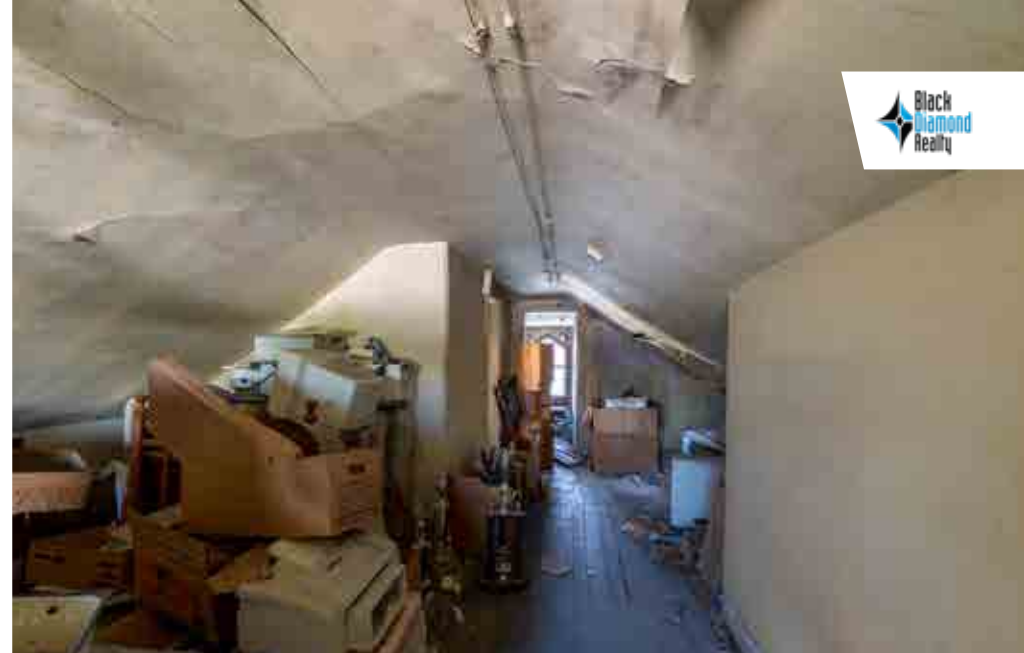
Admin House: Attic/Storage.
