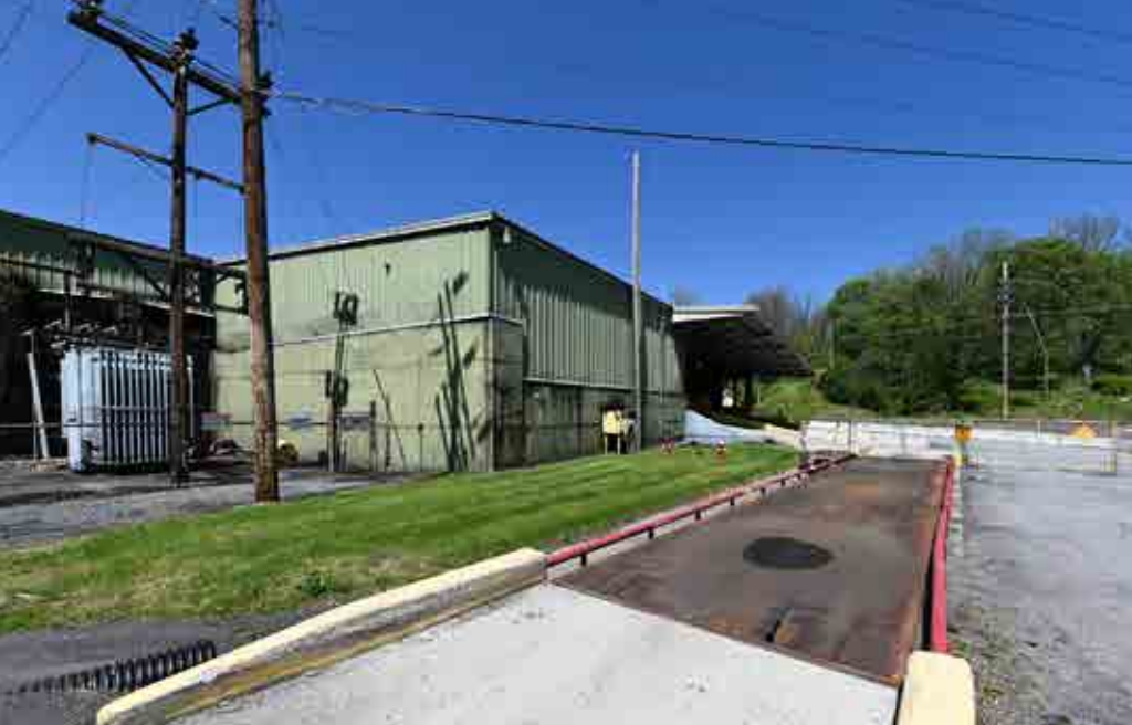
Property Exterior: Zone #5.
