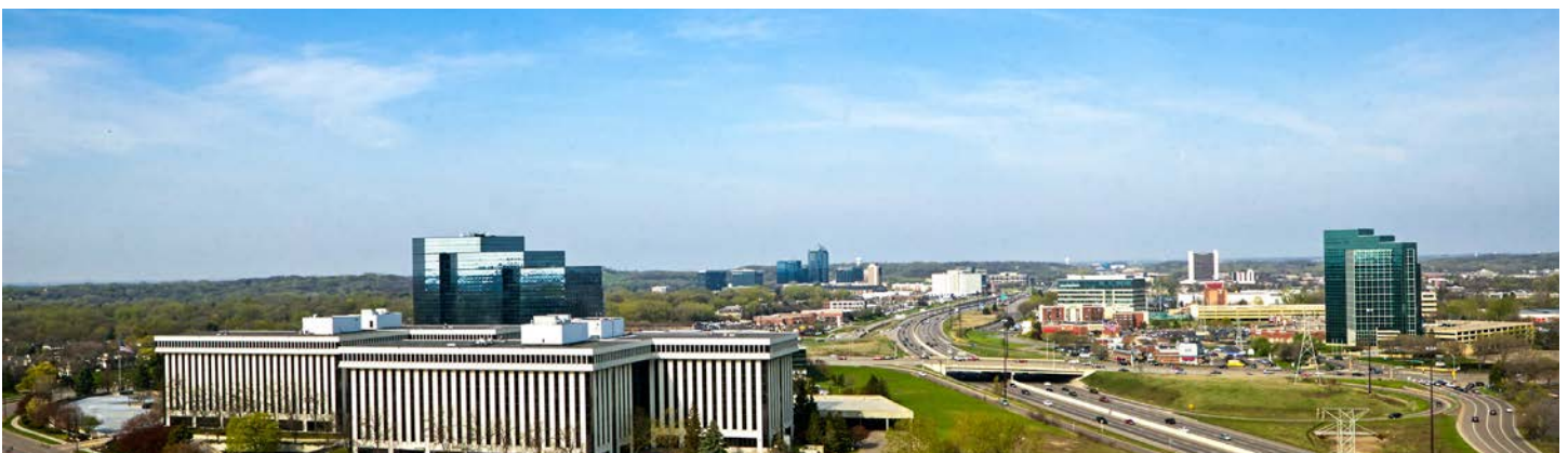
WEST VIEW | TOWARDS INTERSTATE 100
