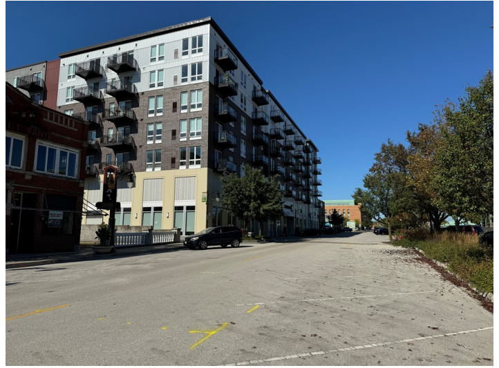
LOCATED NEXT TO NEW MIXED-USE DEVELOPMENT— ELLISON APARTMENTS. BUILT IN 2019.
