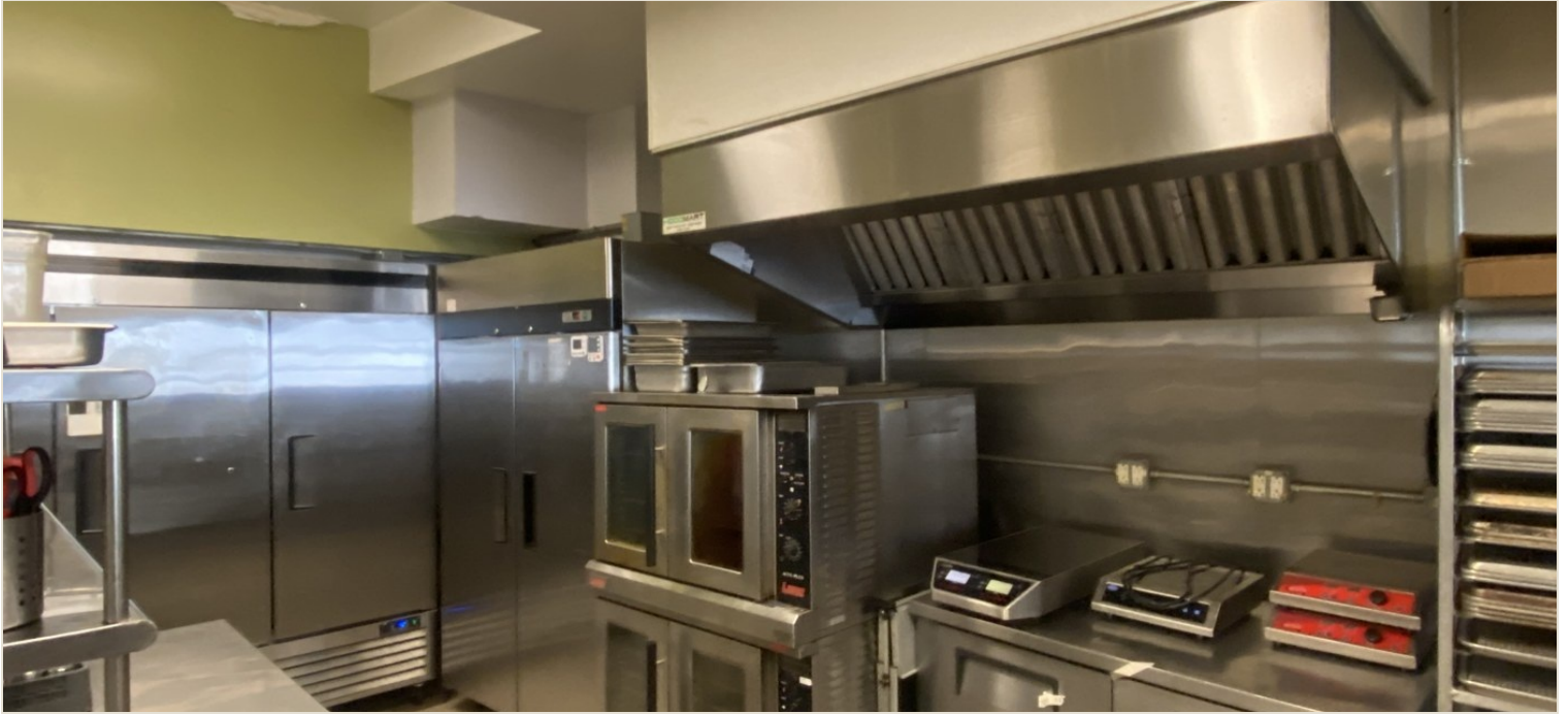
Cook Line — stainless hood system with stacked convection ovens
