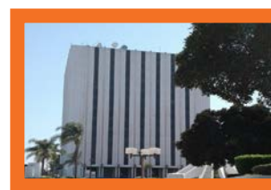
City Hall & Courthouse
