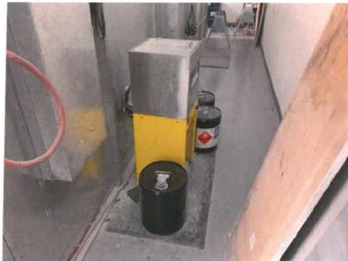
Photo 16: Subject Site (Facing Northeast) First Floor Paint Booth Area
