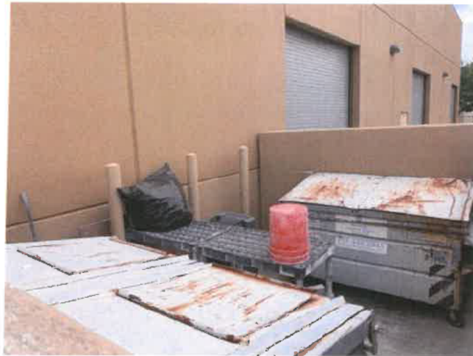
Photo 23: Subject Site (Facing Northeast) Associated Paved Area Trash Enclosure
