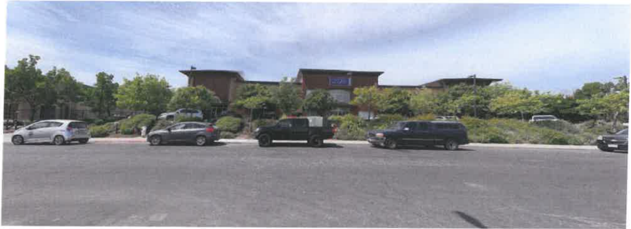
Photo 1: Subject Site (Facing Southwest) Two-Story Light Industrial Building and Associated Paved Areas Along the Southwest Side of Union Way
