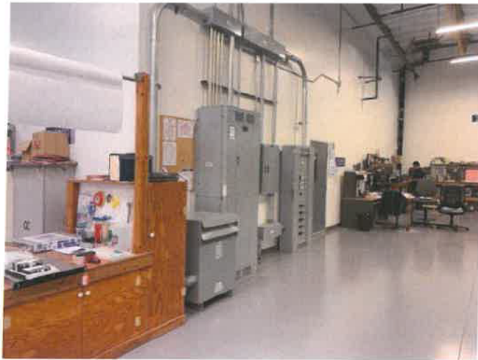
Photo 11: Subject Site (Facing North) First Floor Staging Area
