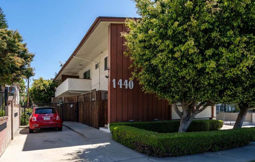
Front of Building
