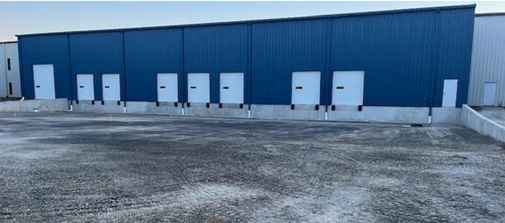
Renovation as of October 2024
