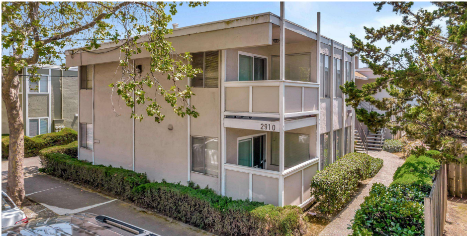
1 2910 Revere Ave Oakland, CA 94605
