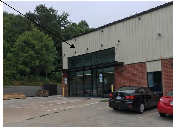
Glass entryway created for tenant. A similar entry can be constructed for space at opposite end of building.
