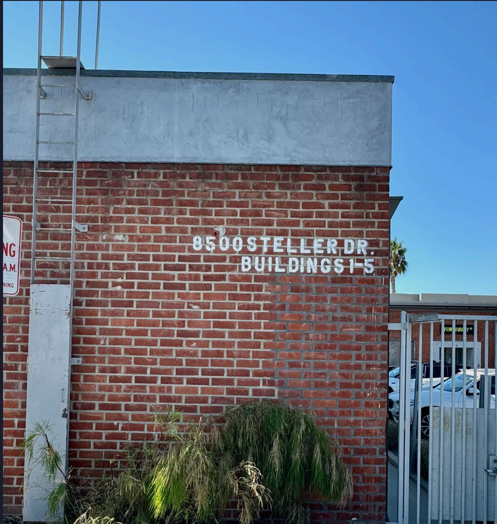
8500 Steller Drive Building 3 / Culver City CA 90230
