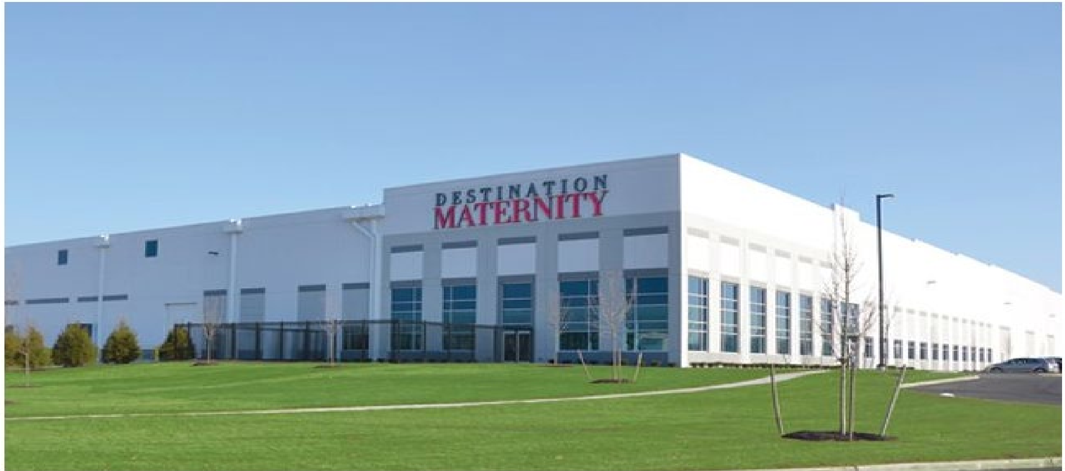
The 400,000-square-foot, built-to-suit facility for Destination Maternity at Whitesell's Haines Center, Burlington and Florence townships.
