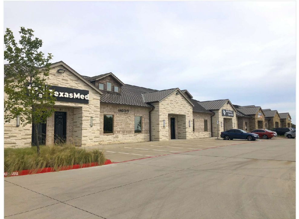
Large Parking area
