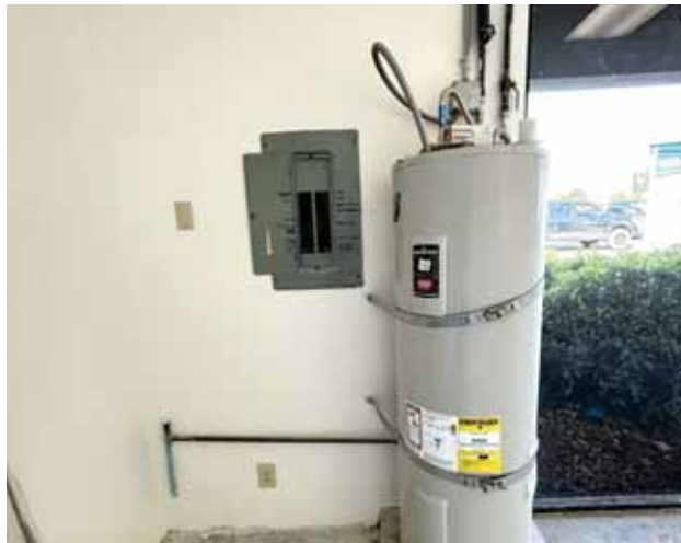
Electrical Panel & 40-Gallon Electric Hot Water Heater
