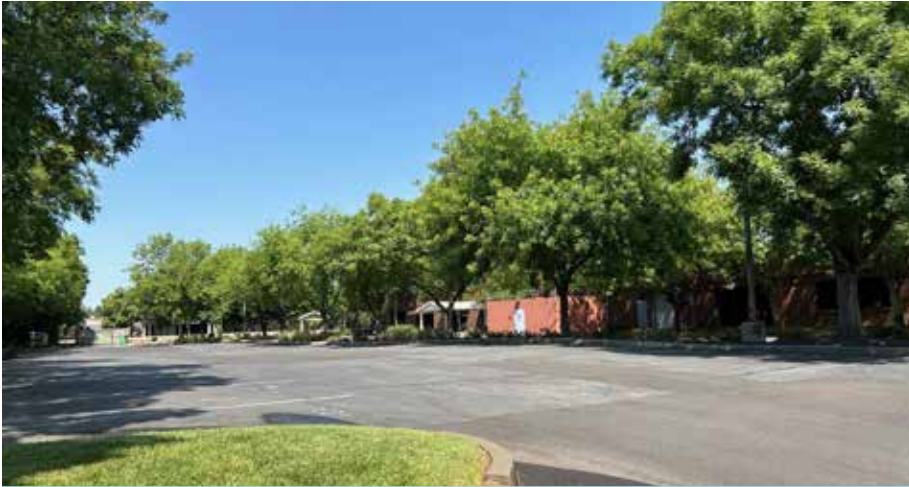
Back of building and parking area
