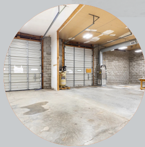
Grade-Level Garage Doors
