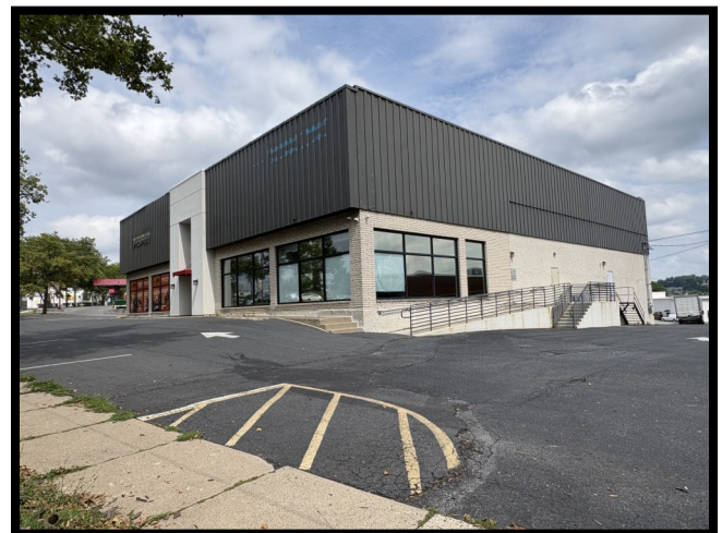
Right side of the building.
