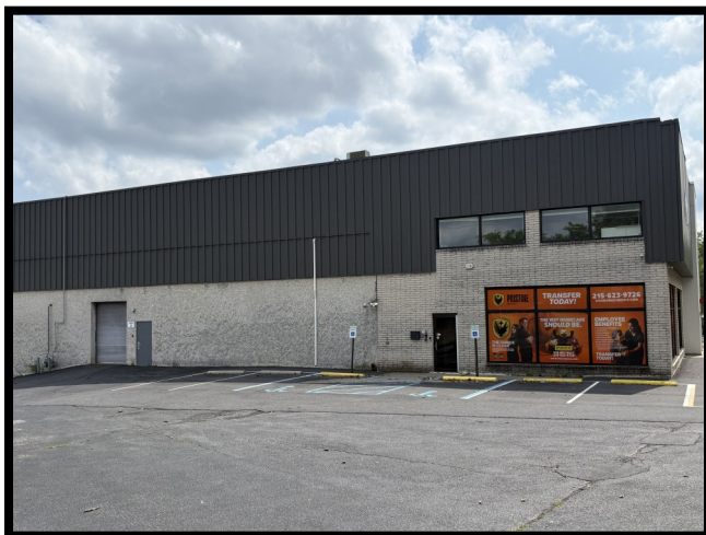
Left side of the building.
