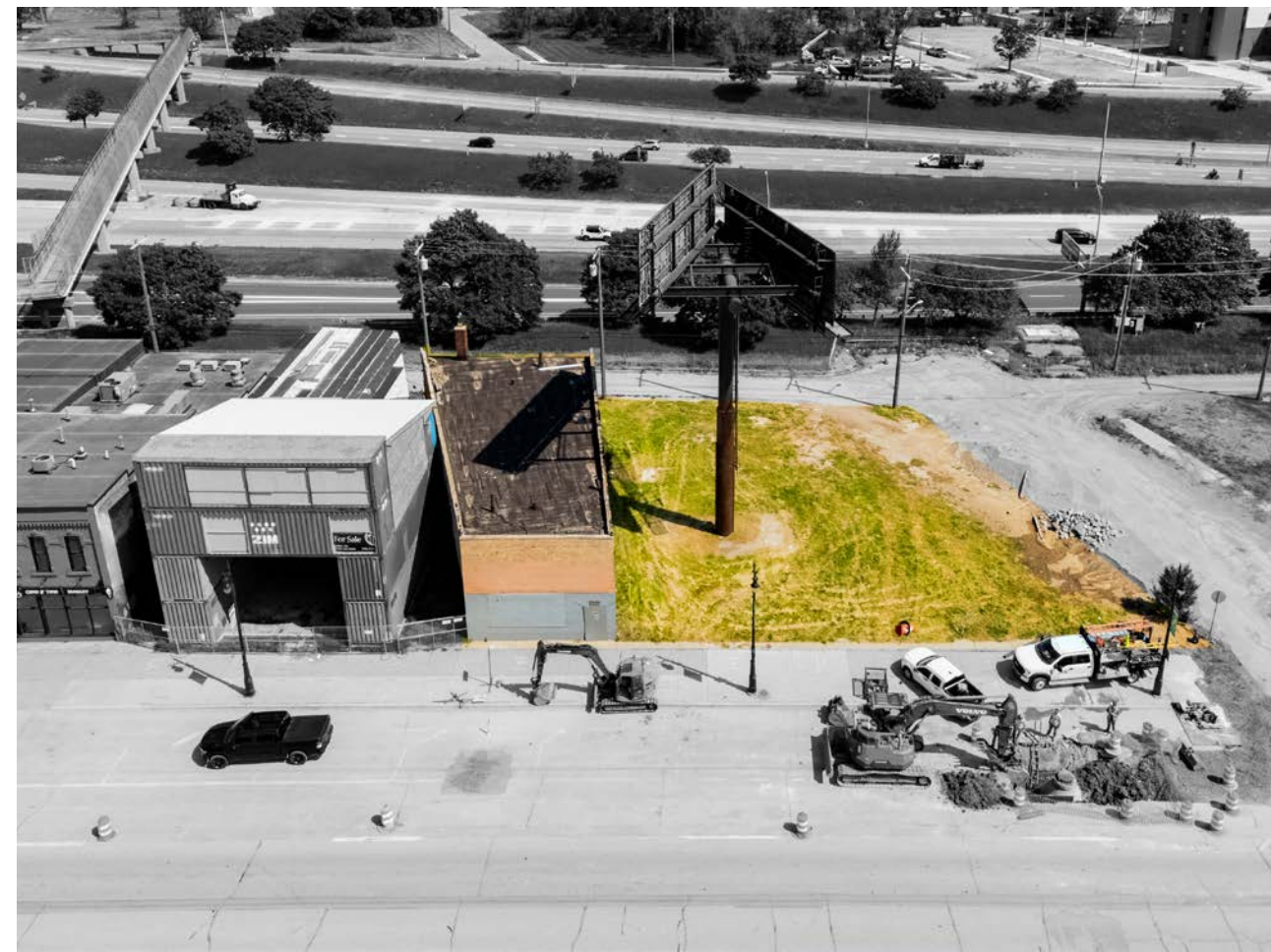
3,000 SF building off Woodward Avenue sitting on a total lot size of 0.292 acres. Includes billboard.
