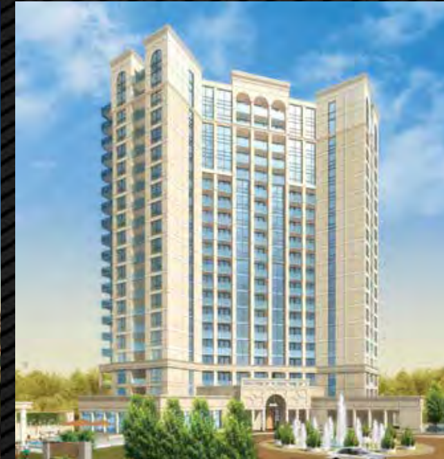
TUSCANY GATES MISSISSAUGA | COMPLETED
