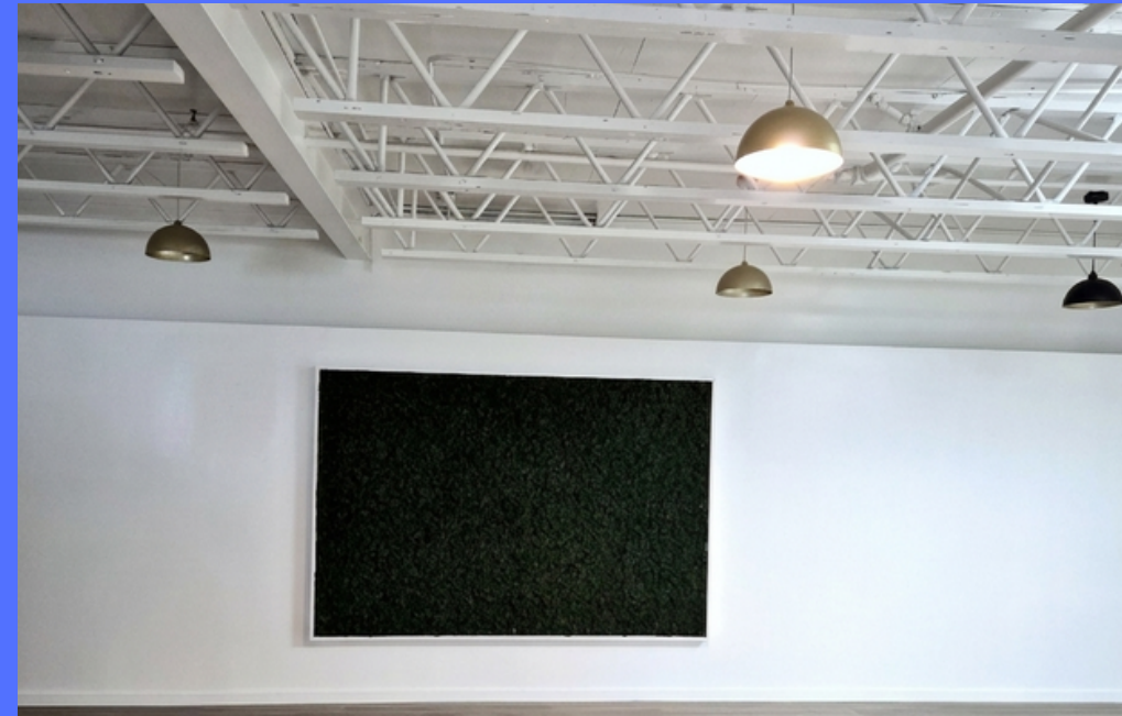
Open work set up
